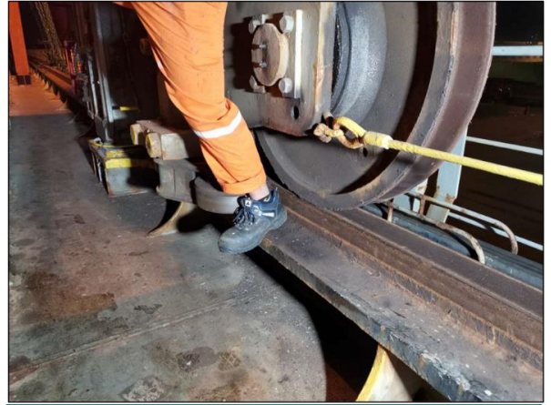
2. The person stepped down on the crane rails, right in front of the crane.
