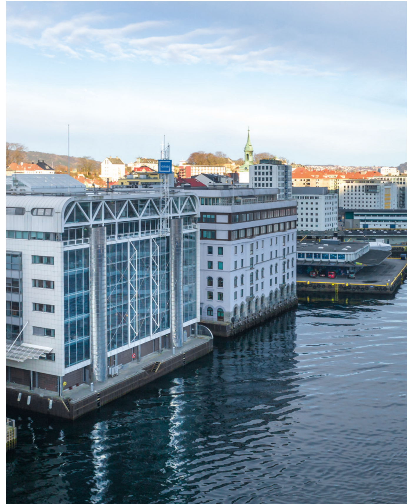
G2 Ocean's headquarters in Bergen, Norway. Photo: Grieg Maritime Group
